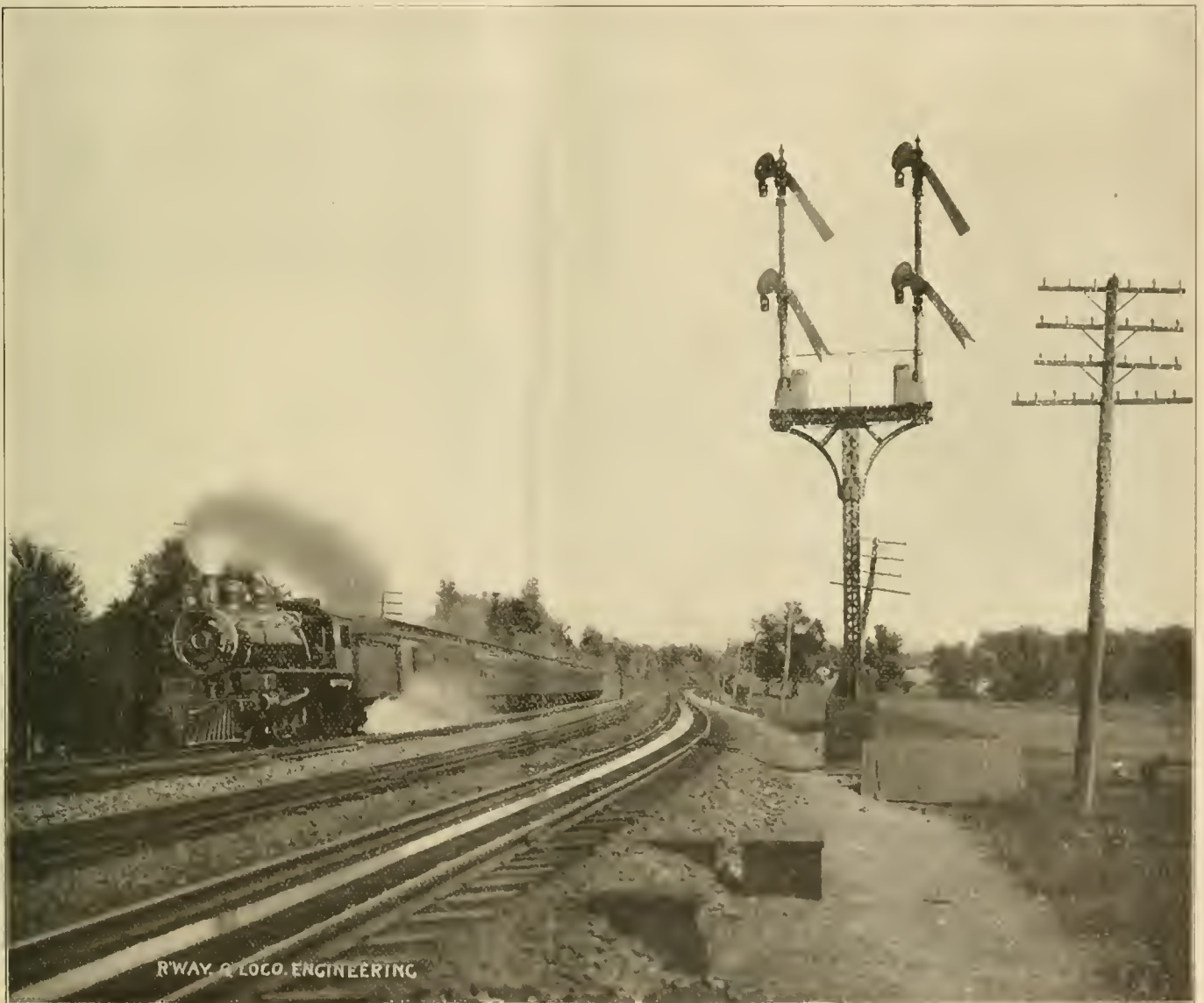
TAKING WATER FROM TRACK TROUGH ON THE P. R. R.
